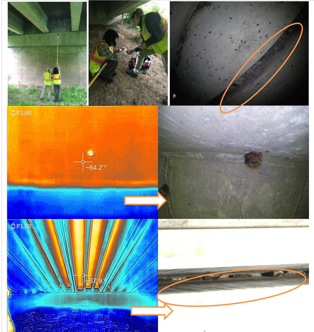
Figure 6. Pictures from field inspections
