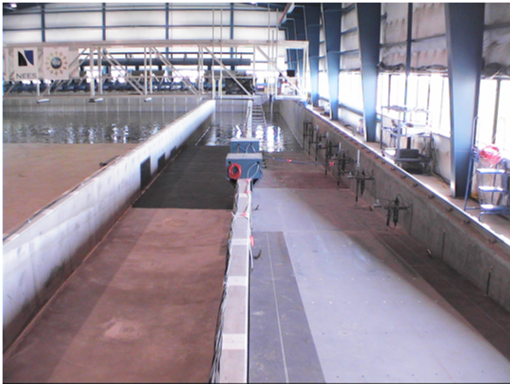
Figure 6.3. Constructed channels in the Tsunami Wave Basin at Oregon State University. (a) View from wavemaker. (b) View from end of channels.
