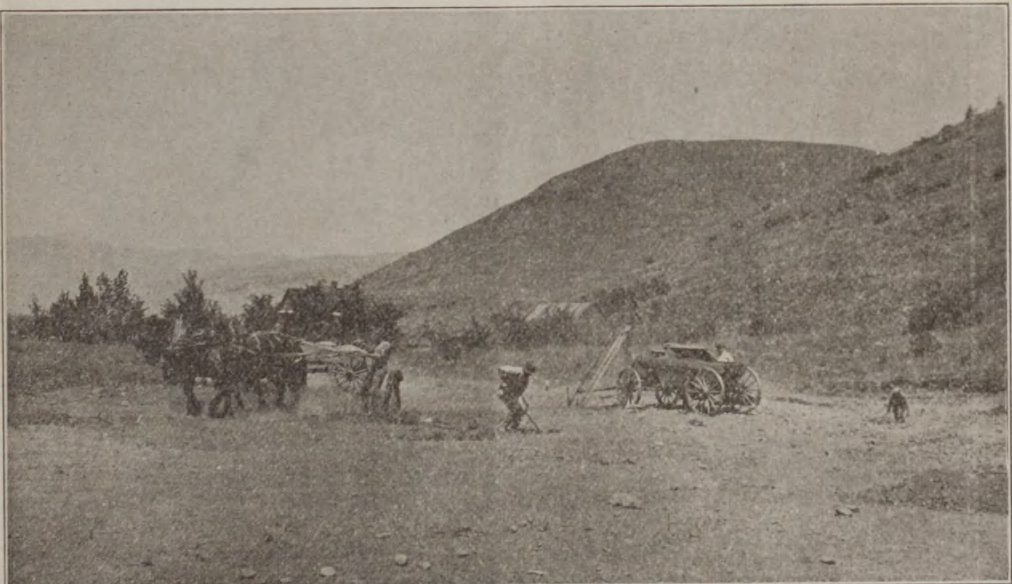
Student Labor Employed in New Field Construction.
