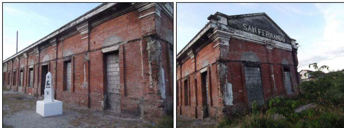
Figures 100 and 101: Exterior views of the San Fernando train station (July 2011).
