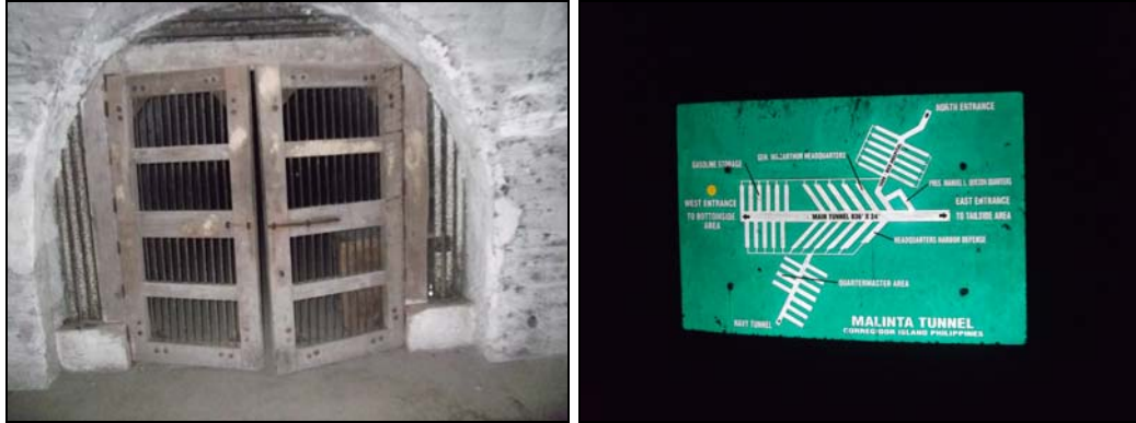
Figures 50 and 51: Entrance to one of the peripheral tunnels on the north side (left); map of the Malinta Tunnel complex (right), Isla ng Corregidor (July 2011).
