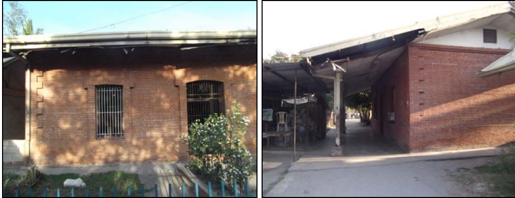
Figures 94 and 95: Exterior views of the Capas train station (July 2011).
