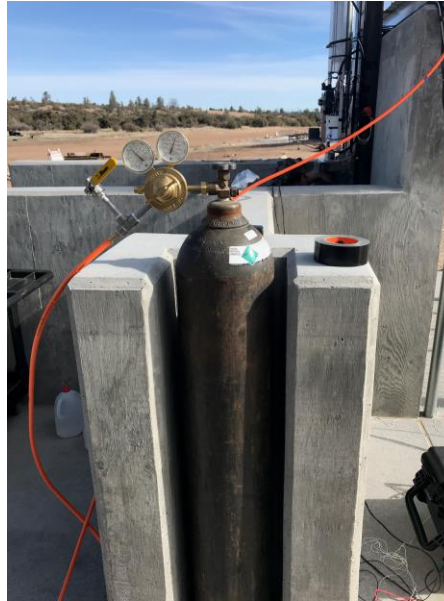
Low pressure GN2 for pneumatics
