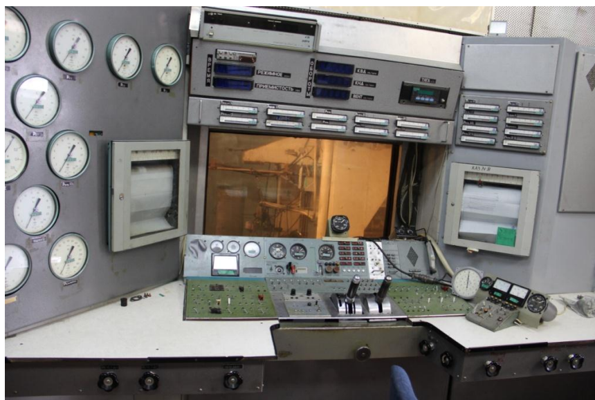
Fig. 6.6. Control room for engine’s operation control during the tests
