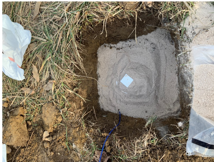
Figure 4.9: Installed Sensor Before Full Burial
