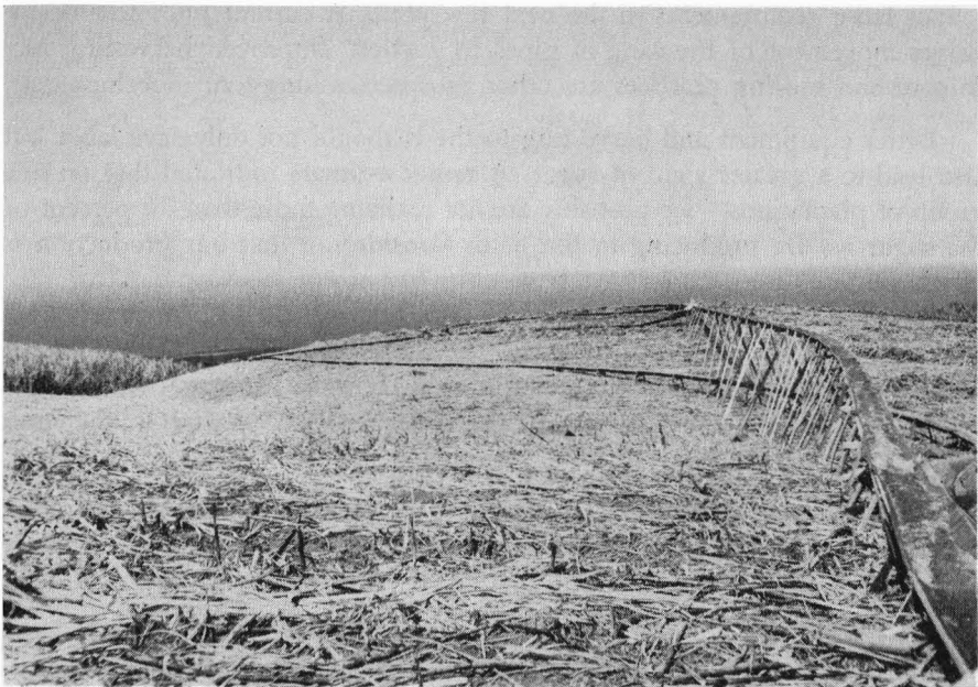
FIGURE 14. Flumes: water was used not only to irrigate the land but to carry harvested cane to the mill.
