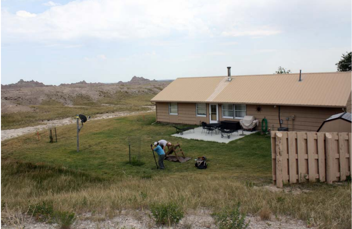
Figure 13. Overview of the shovel test area at Quarters 29. Laura Bender and Allison Young excavate shovel test 1 in advance of fence installation.
