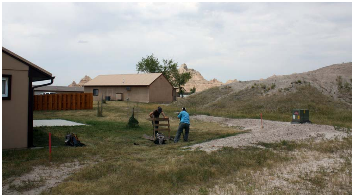
Figure 12. Overview of shovel test area in advance of privacy fence installation at Quarters 28. Erin Dempsey and Laura Bender excavate shovel test 1.
