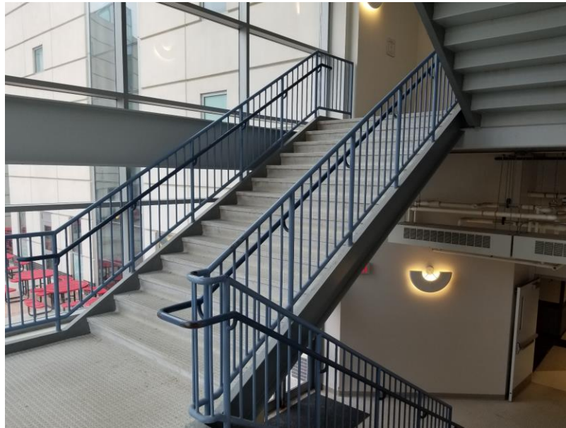
Figure 2.4: Stair Case Structure Used in Study
