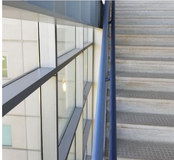
Figure 3.10: Glass Façade Curtain Wall
