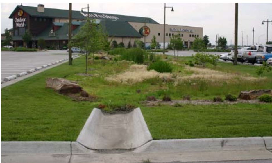
Below: Vegetated drainage swale between parking lots at Bass Pro Shops in Council Bluffs, Iowa. (Photos courtesy Steve Rodie)
