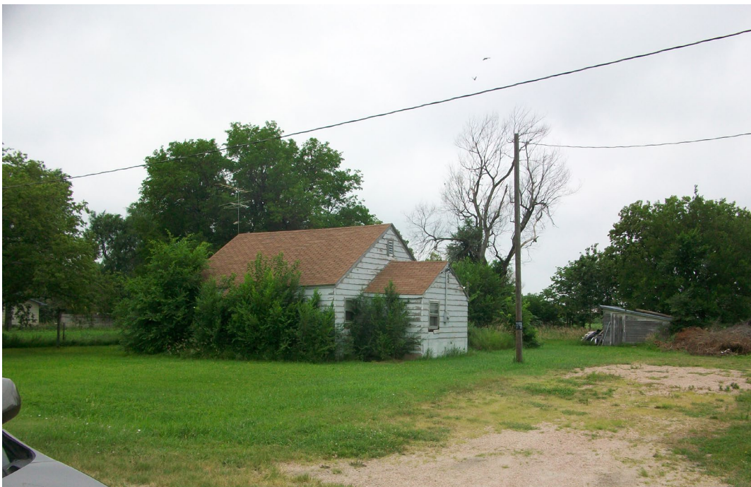
Figure 5.14. Grand Island Farmsteads. This is Homestead “H” as it appeared during a site visit in 2014. The small structure to the right of the house appeared to be a chicken coop (Glanz, 2014).
