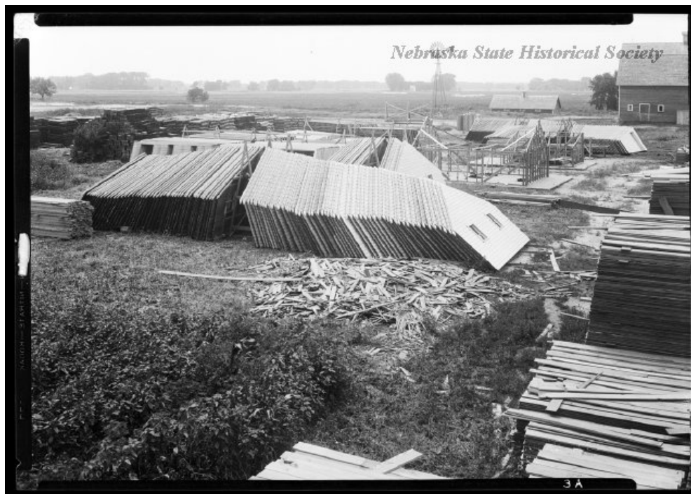
Figure 5.27. Two Rivers Farmsteads, 1935. “Prefabricated materials for more than 50 structures are stacked together in this farmyard” (Nebraska State Historical Society).
