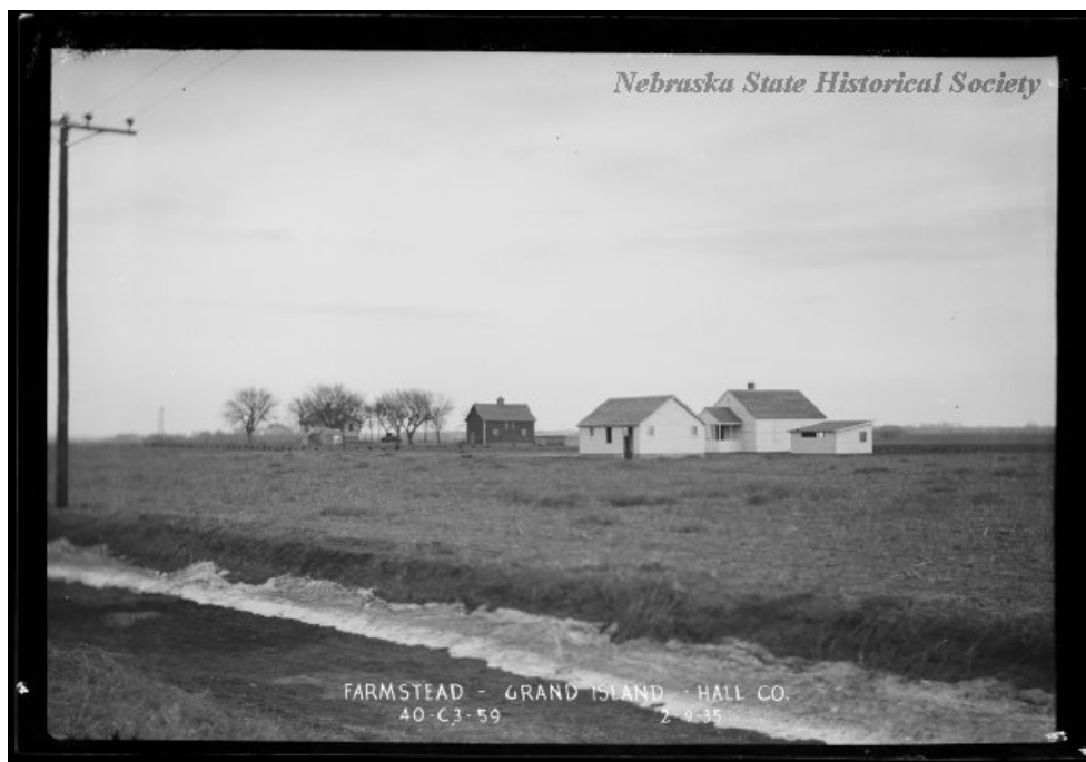
Figure 5.10. Grand Island Farmsteads, 1935. New construction (house, chicken coop, and garage/cow barn) is in the foreground. Existing buildings in the background were purchased with the land. View is from Highway #2 looking northeast (Nebraska State Historical Society).
