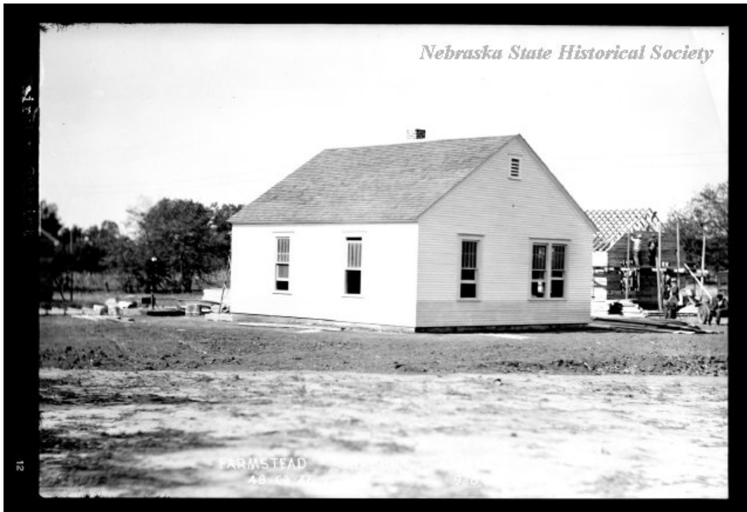
Figure 5.7. Fairbury Farmsteads, 1934. House under construction (Nebraska State Historical Society).
