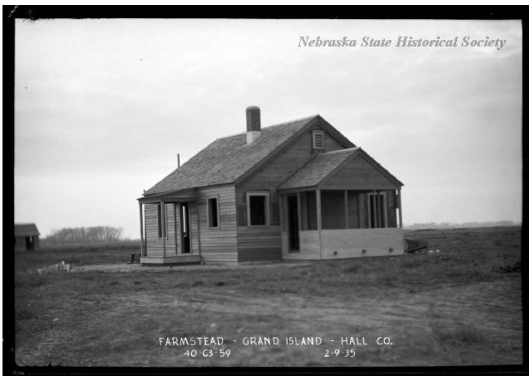
Figure 5.15. Grand Island Farmsteads, 1935. House is under construction. The structure in the center left of the picture is a garage/cow barn of another subsistence farmstead (Nebraska State Historical Society).
