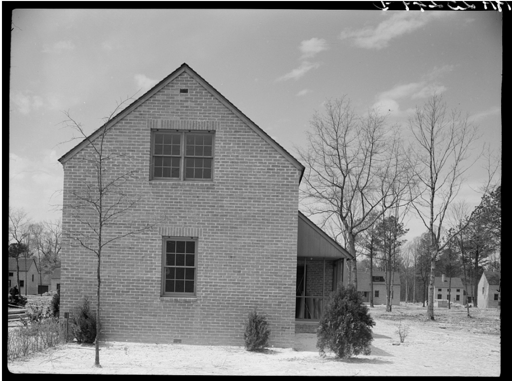
Figure 4.4. One of the completed homes in the Newport News Homesteads community (Rothstein, 1937).
