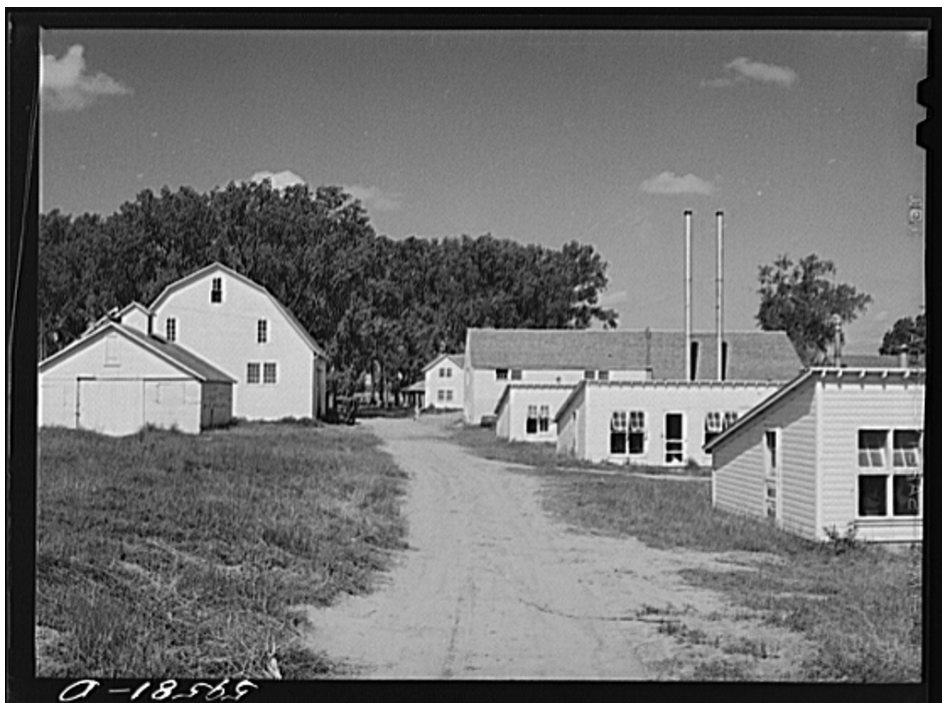
Figure 5.29. The barns and chicken coops are part of the cooperative buildings at the Two Rivers Farmsteads. The house at the end of the road (center) is the cooperative's community building (Wolcott, 1941).
