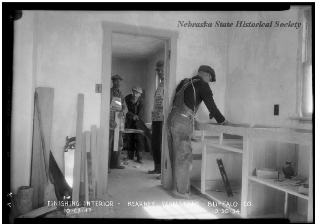
Figure 5.32. Constructing kitchen cabinets for a Kearney Farmsteads home, 1934. (Nebraska State Historical Society).
