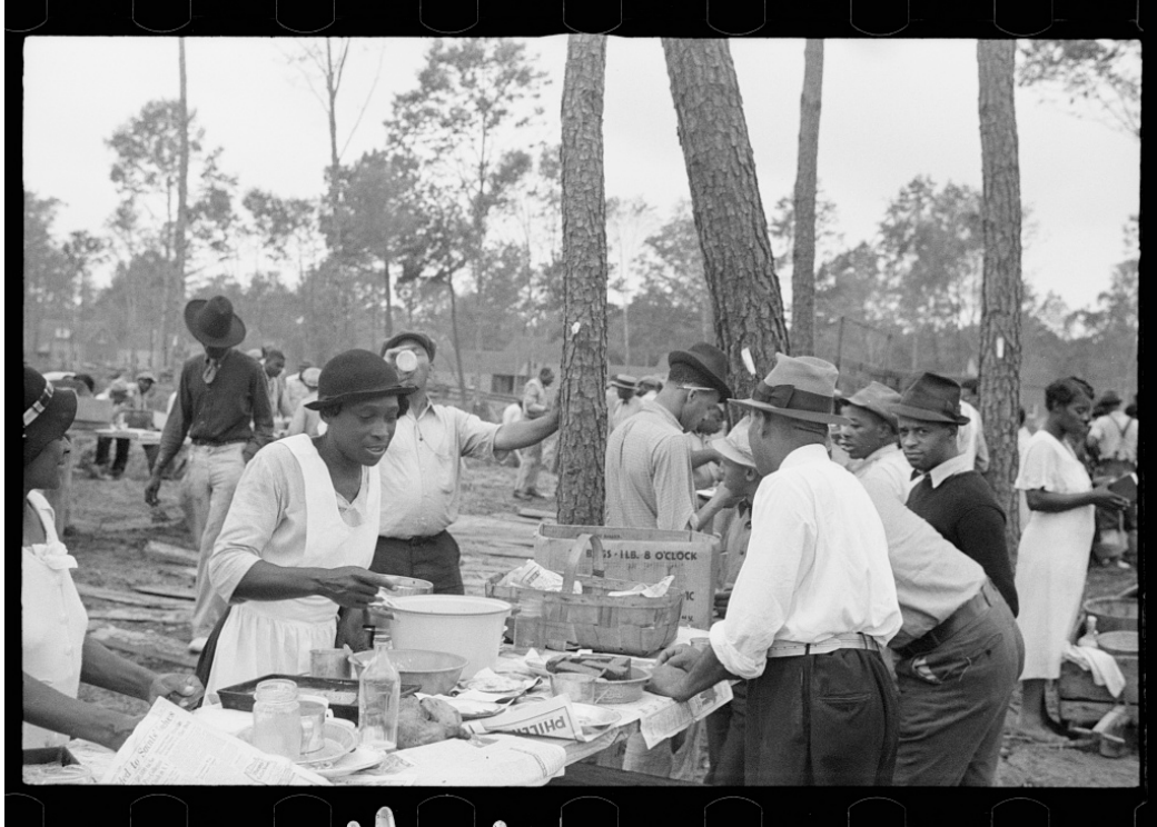
Figure 4.3. Serving lunch to the workers during the construction of the Newport News Homesteads (United States Resettlement Administration, 1936).
