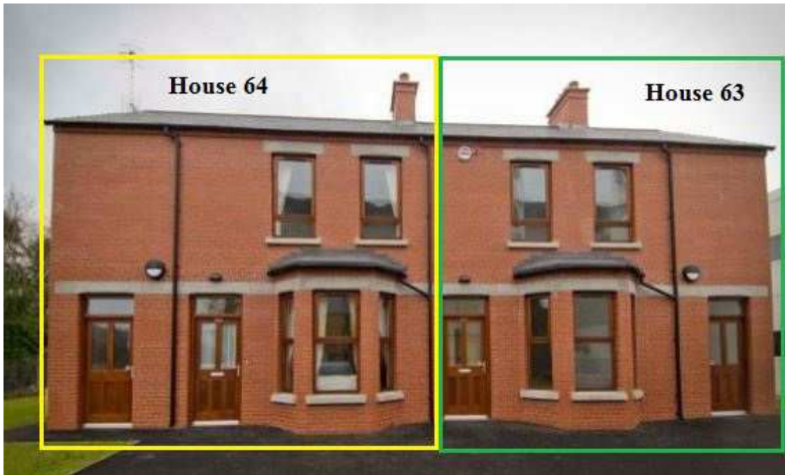
Figure 2: Two mid-terraced houses used for testing the retrofit CAWHP heat pump.
