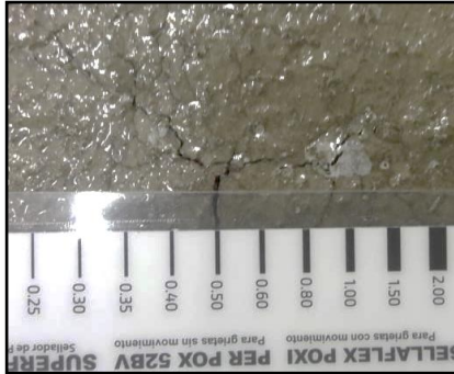
Figure 4. 0.50mm fissure.
