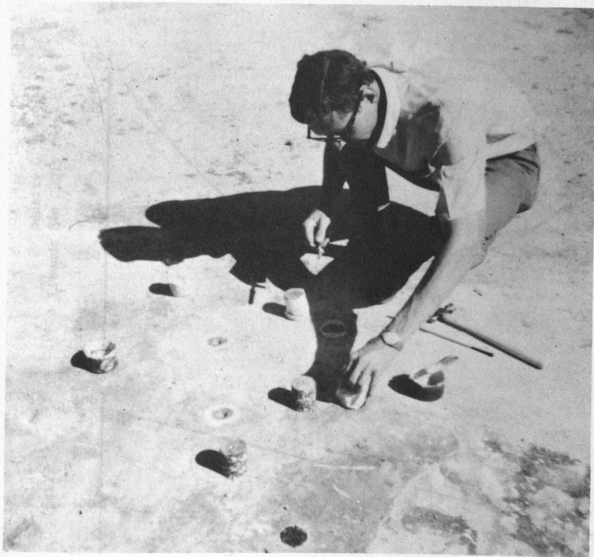
Figure 9. Placing Couplings in the Inspection Holes
