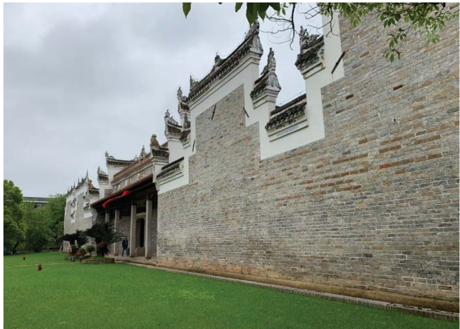
Figure 6.9 Western facade of academy
