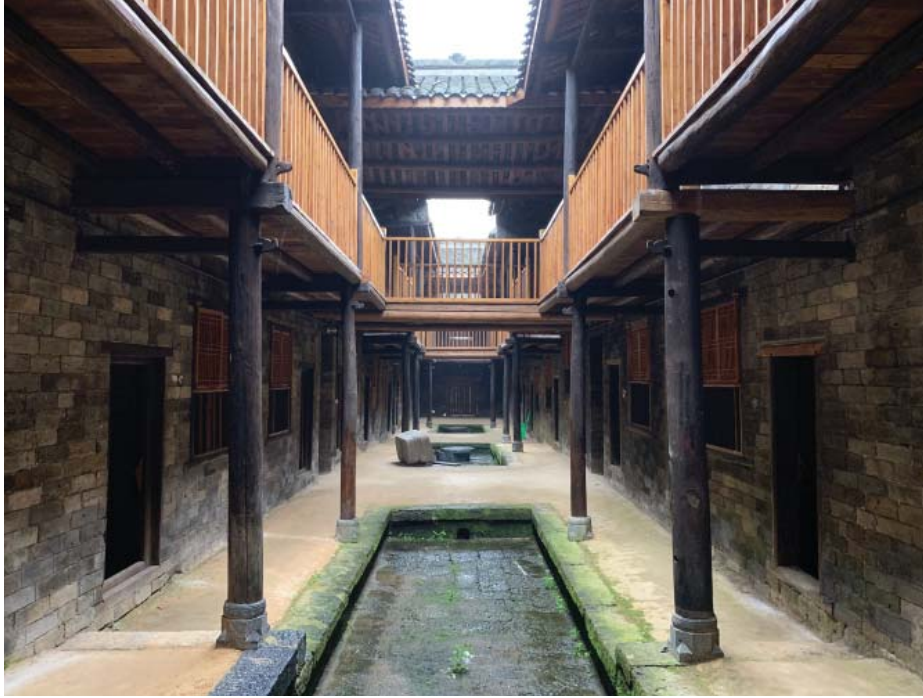
Figure 5.7 View of standard linear Tian-jing courtyard, similar spatial porportion for eight centre rows.
