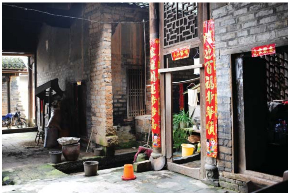
Figure 1.5 A side chamber next to a linear Tian-jing. Various household furnishing populated the space, and the door of the unit was left open.
