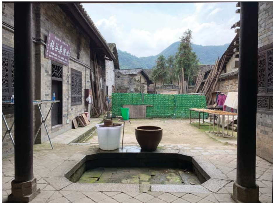
Figure 4.10 Void space left from the deconstruction of the outer sections of the second west branch house
