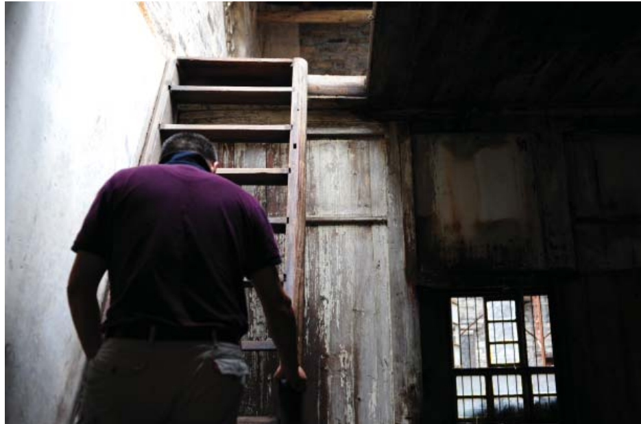
Figure 1.16 Original wooden stairs in one of the chambers under restoration
