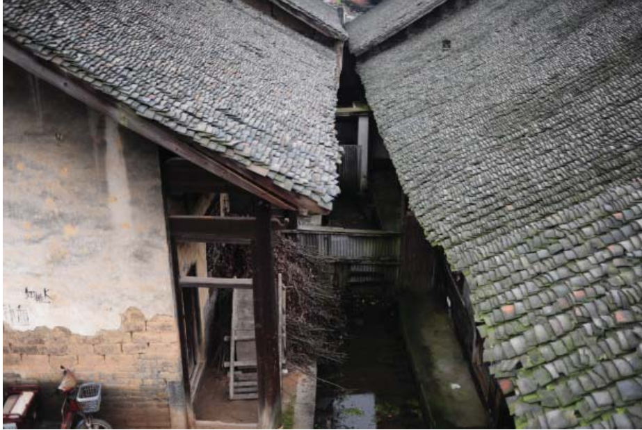
Figure 1.10 Looking down from the flat roof platform, seeing the linear Tian-jings connecting the rows of buildings together
