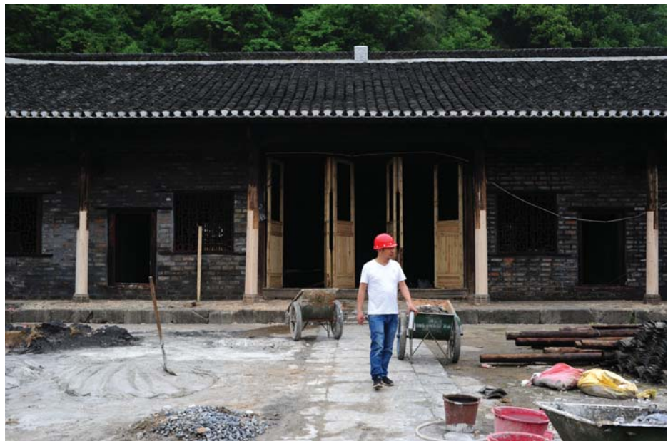
Figure 1.21 Left: Upper Main House under restoration
