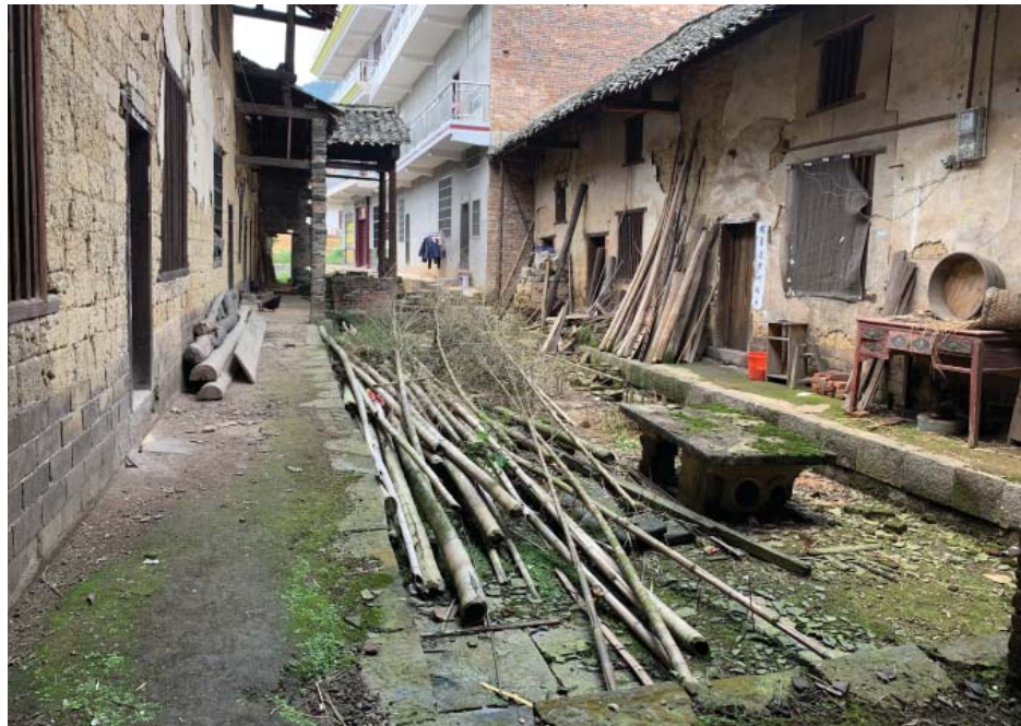
Figure 2.7 Rear side Tian-jing, compound beyond courtyard had been rebuilt
