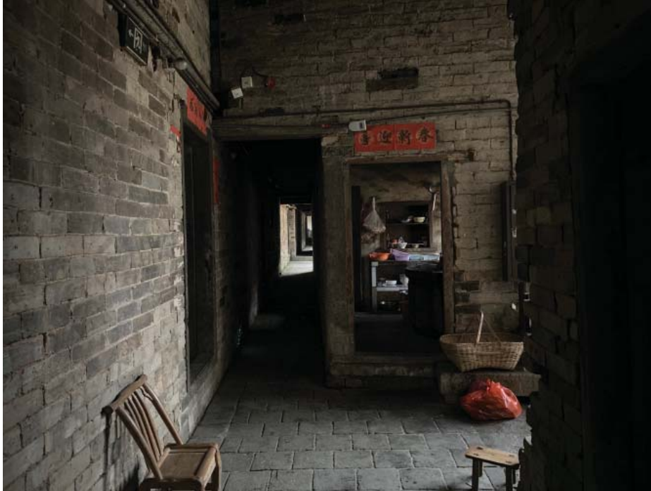
Figure 4.14 Kitchen set up next to the west transverse corridor for convenience of dining service along the main house.
