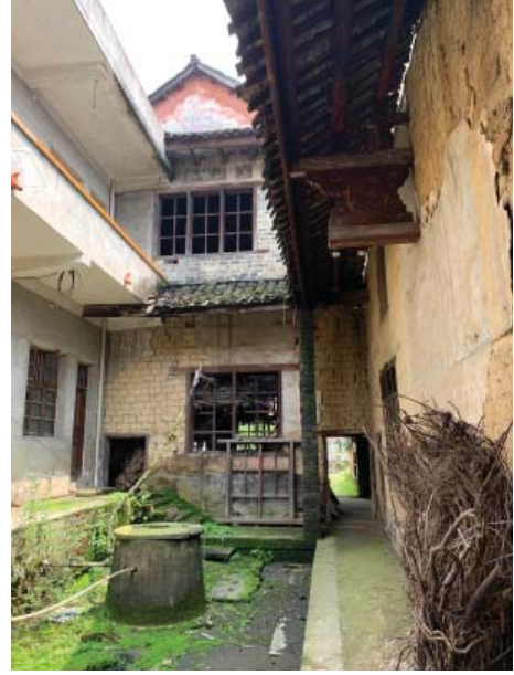
Figure 2.13 Central tower of Perpetual Progeny Hall, side entrance
