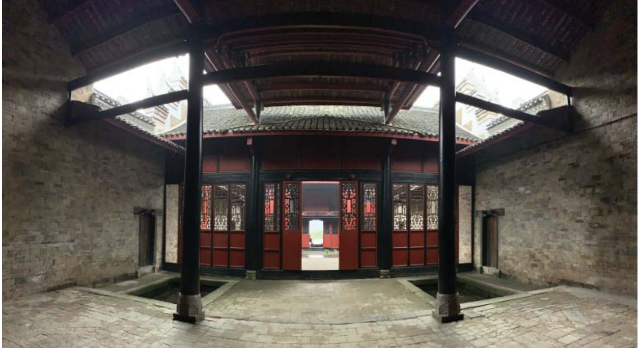
Figure 5.3 Interior view of double Tian-jing openings and connecting air tower in the second jin of the ancestral hall from the north
