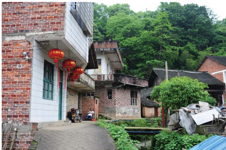
Figure 1.14 Modern private constructions between the Longxi mountain, the original compound walls, and the Longxi stream.
