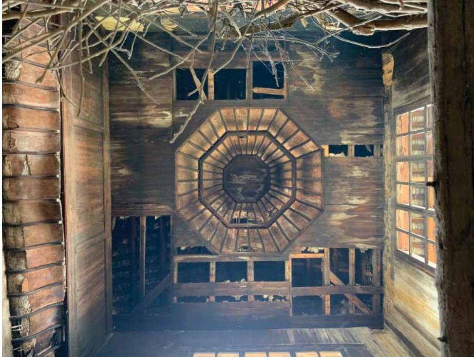
Figure 2.14 Intact octagonal ceiling finish within the tower of the Perpetual Progeny Hall, windows on three sides of the tower
