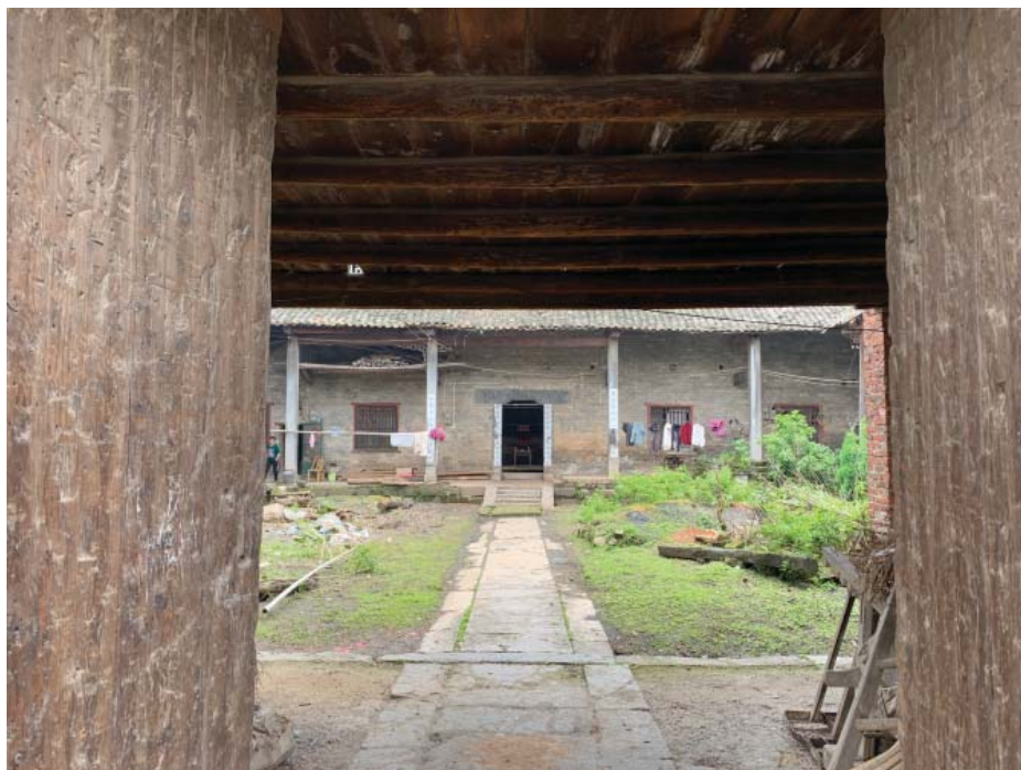
Figure 2.8 View of the Greater Teaching Hall from the front gate
