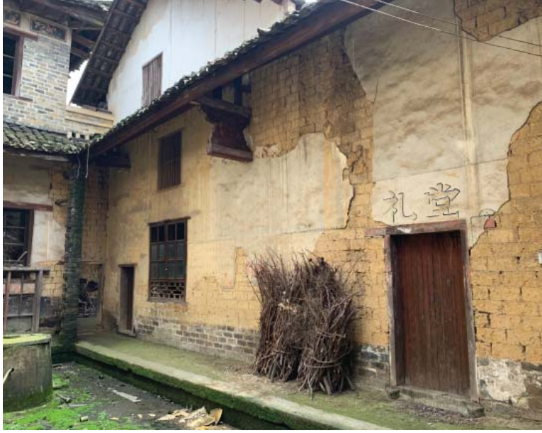
Figure 2.12 Wall Paint peeled off to show the brick structure behind
