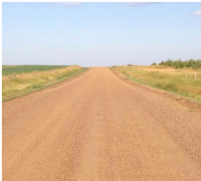
Figure 2.10 Gravel road with adequate crown.
