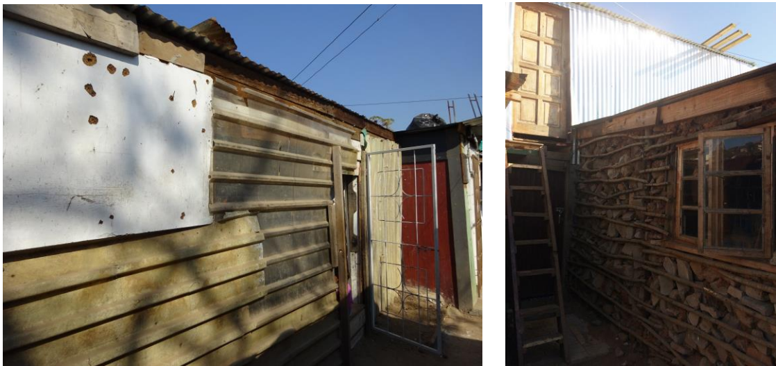
Fig.35 & 36: The image on the left depicts the typical wooden frame structure type of dwelling clad in a mixture of materials in the Quarry Road West Settlement in Durban, South Africa. The image on the right however depicts a much more developed dwelling of more robust construction, whose residents have been in the settlement for much longer. (Source: Author)
