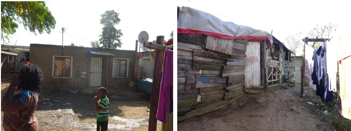
Fig.66: Image of a dwelling in Quarry Road West showing brick construction plastered over – depicting permanence (Source: Author)
