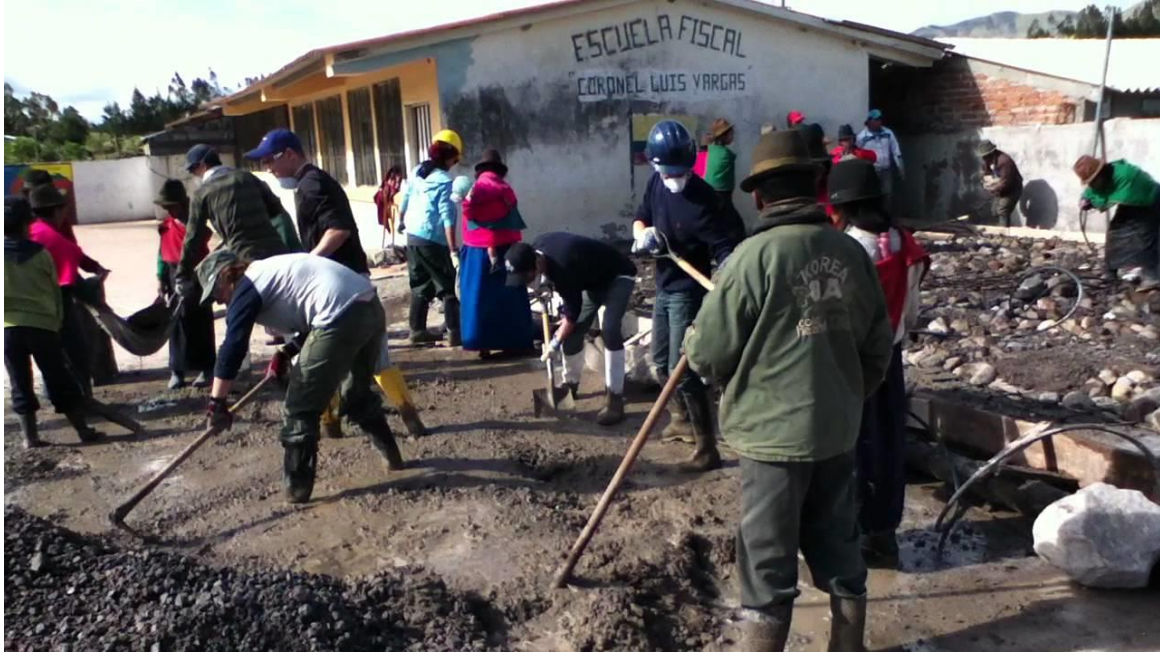
Fig.12: The above image depicts the way the community in an Ecuadorian informal settlement work together to complete one of the resident's dwellings. An adaptation of the Minga ceremony of raising the roof of the traditional dwelling in a rural setting to now, in an informal settlement with a concrete roof and motivated by financial reasons to avoid using professional labour.
