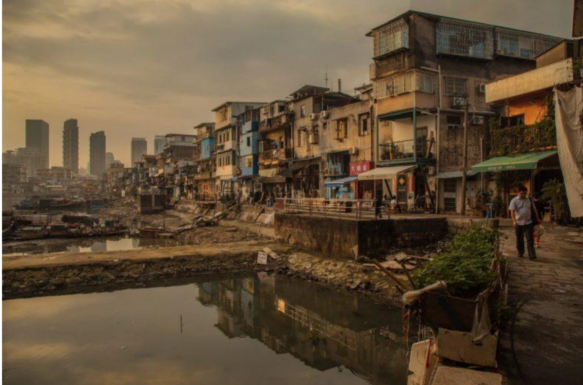
Fig.23: A row of dwellings in an informal settlement in Mumbai displaying contrasting degrees of completion, creating a heterogeneous spectacle.
