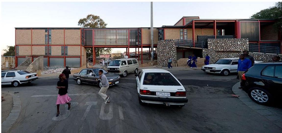
Fig.108: The north façade of the building showing the large expanses of brick infill which was produced locally and built into the façade by the community. (Source: Baan, 2010)
