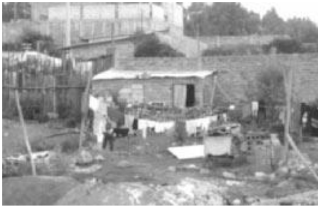
Fig.13: The above image is of a typical Mediagua dwelling with block walls and a corrugated iron roof. (Source: Klaufus, 2001)
