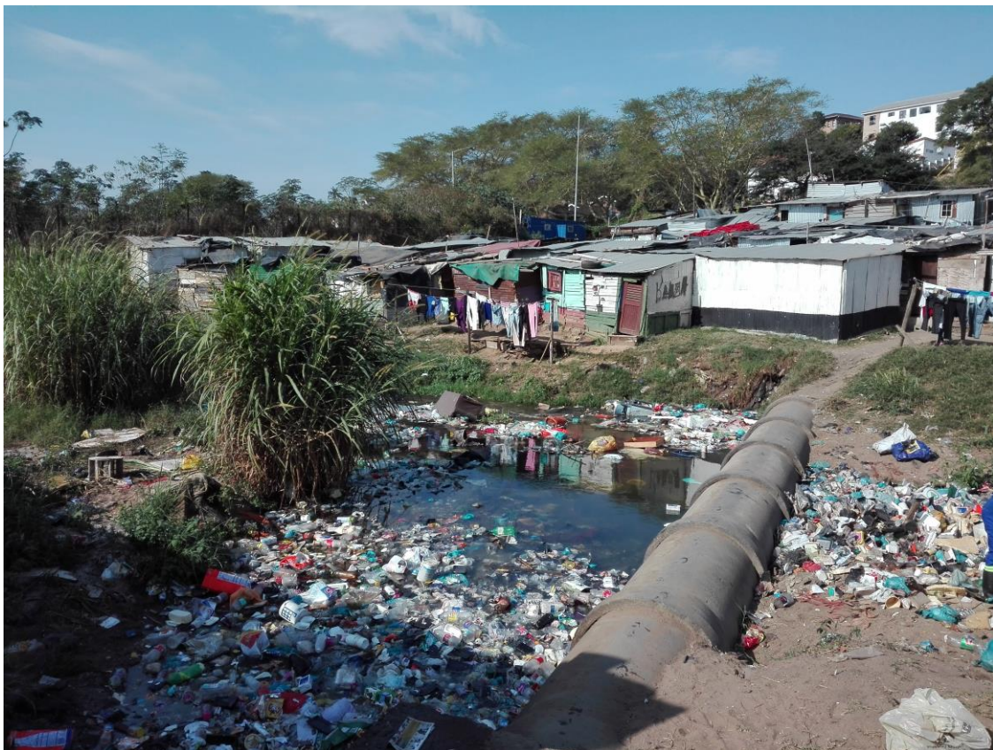
Fig.74: The polluted Palmiet River that runs through the Quarry Road West Informal Settlement poses a major health and safety issue (Source: Author)
