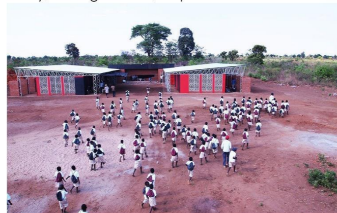
Legson Kayira Community Centre Mchinji, Malawi Architects for A Change
