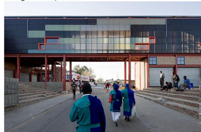
Alexandra Interpretation Centre Alexandra, Johannesburg Peter Rich Architects
