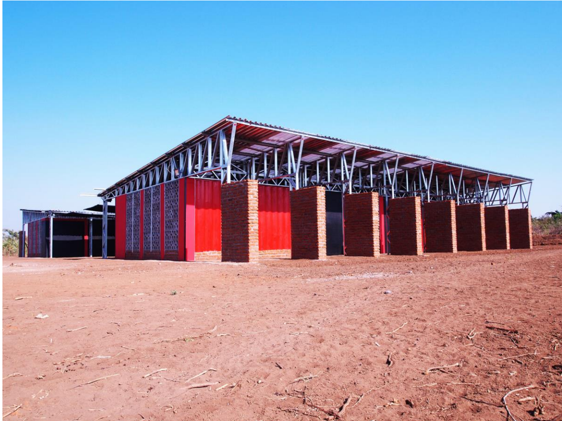
Fig.115: An exterior view of the building showing the assortment of materials used in the buildings construction. From the high tech frame structure to recycled shipping containers and breeze blocks. (Source: Archdaily, 2014)
