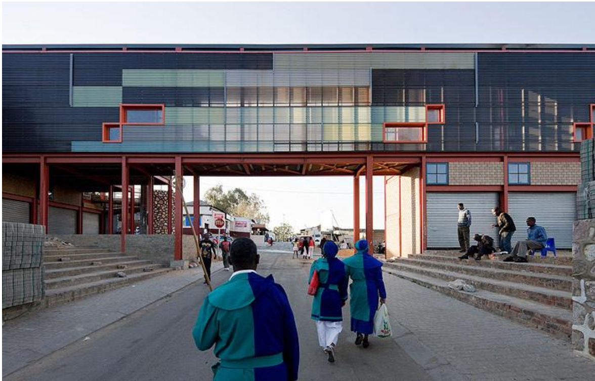
Fig.109: The main exhibition space composed of an assortment of corrugated metal and polycarbonate sheeting and the contrasting brickwork all infilled into the steel frame structure.
