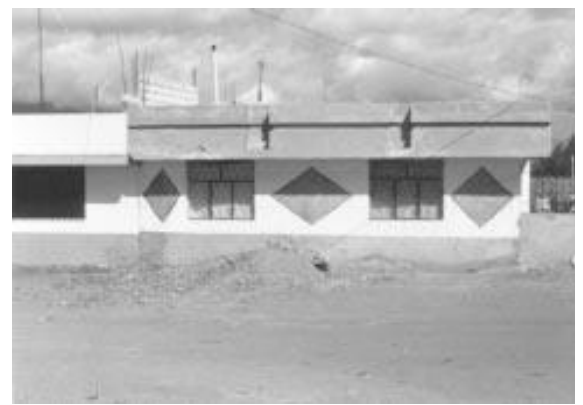
Fig.14: Depicts a typical Casa dwelling with plastered block walls and a concrete roof. (Source: Klaufus, 2001)
