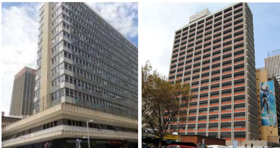
Figure 2- 4 inner-city dilapidated building and on converted into public housing (Johannesburg Social Housing Company, 2012)
