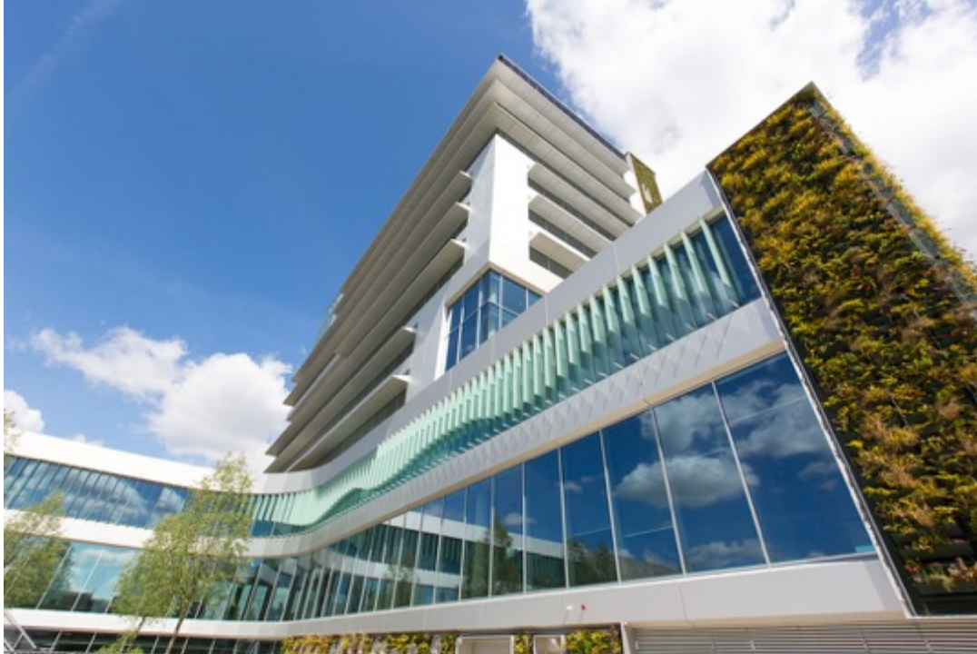
FIGURE 10 TECHNOLOGICAL SOUTH FAÇADE INCLUDING ENERGY PRODUCTION
