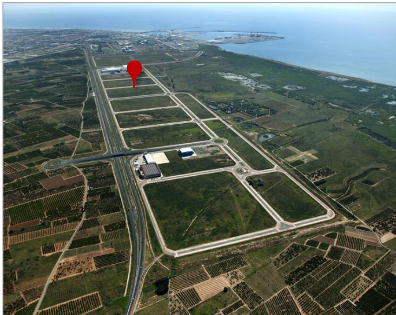
Figure 1. Aerial view of the Parc Sagunt I land plots. [3]
