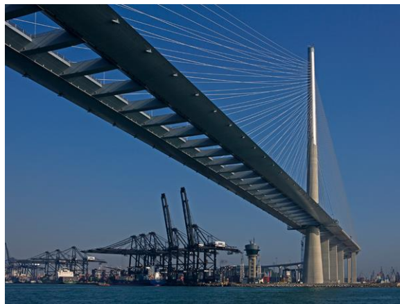
Figure 6. Stonecutters Bridge (word-architects.com)
