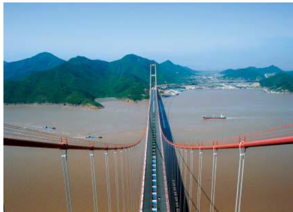
Figure 5. Sihoumen Bridge (china.bridge.org.cn)
