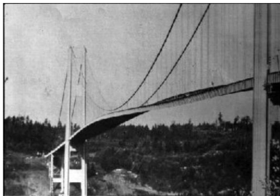
a) First Tacoma Narrows Bridge ( www.txstate.edu )
