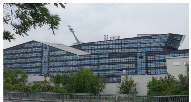
Fig. 5 - T-Mobile Austria building, architectural abstraction of a cruise ship with considerable static requirements and dead space because of the contrast between the inner and outer structure of the building (Vienna, Austria; G. Weiss).
