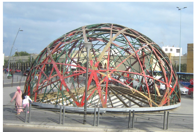
Fig. 13 - Modern coffee cans, (above); half spherical cover over an underground bus station, Marrakesh, Morocco. (G.Weiss).
