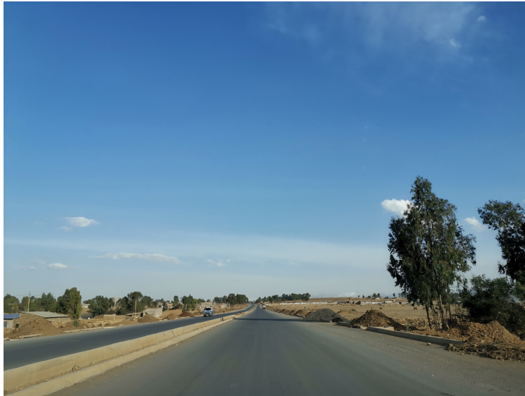
The industrial park is located outside of Mekelle. Photo by Istvan Tarrosy.
