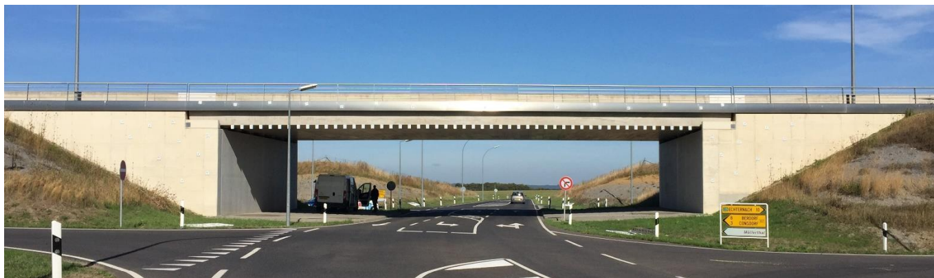
220 Figure 4. The experimental bridge in Altrier in Luxembourg
