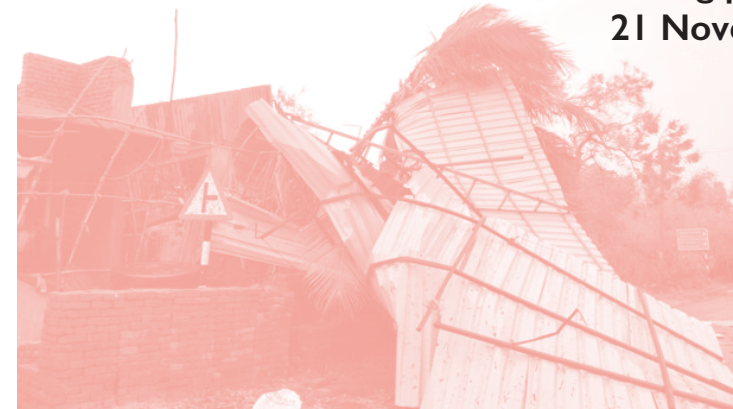
Image 20. Site of destroyed houses due to cyclone Image credits © BBC
