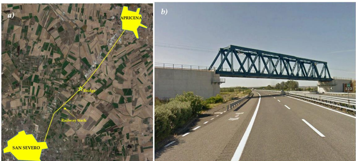
227 Fig. 1 – Geographical framework of the test site (a) and the truss bridge overpassing the “A14” Italian motorway (b)
