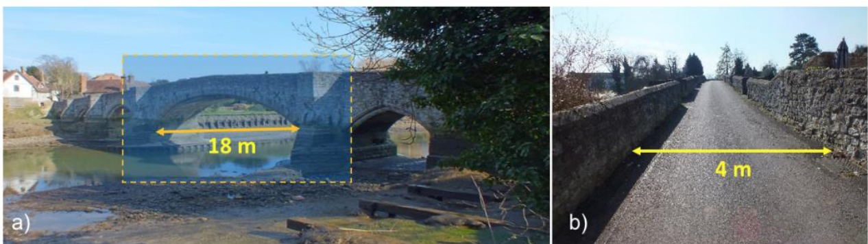
350 Fig. 4 Main features of the “Old Bridge” at Aylesford in Kent, UK. (a) side view of the bridge spans with 351 details of the main central arch span width and (b) width of the carriageway.
