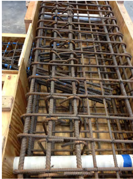
Figure A.3 - Bottom block reinforcement inside formwork
