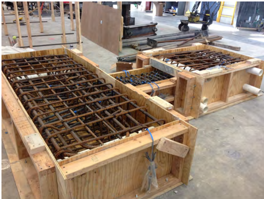
Figure A.6 - CB2 before casting
