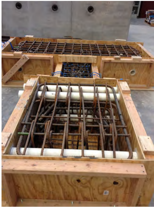
Figure A.5 - CB1 before casting
