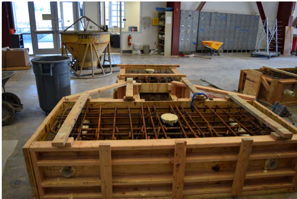
Figure A.8 – CB2AD before casting (steel pipes embedded into top and bottom blocks)
