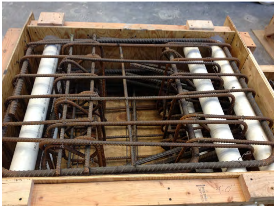
Figure A.4 - Top block reinforcement inside formwork
