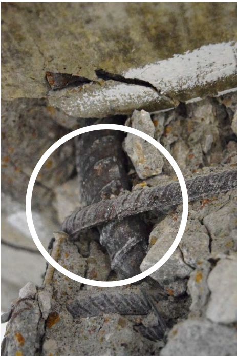
Figure B.22 – CB1 with diagonal bar buckling during first cycle to -6% chord rotation
