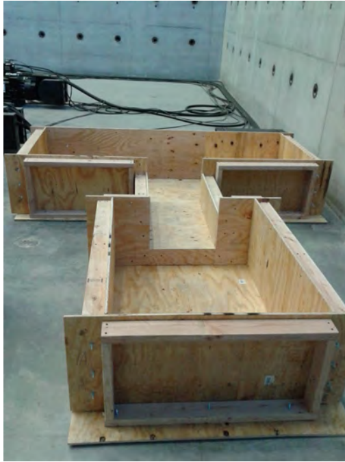
Figure A.1 - Formwork for a coupling beam specimen
