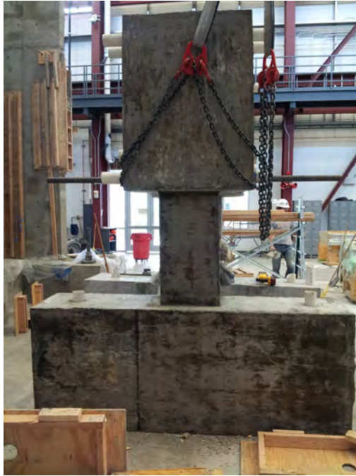
Figure A.11 – Coupling beam specimen after stripping formwork
