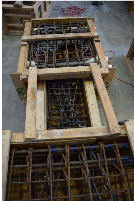
Figure A.9 – CB3D before casting
