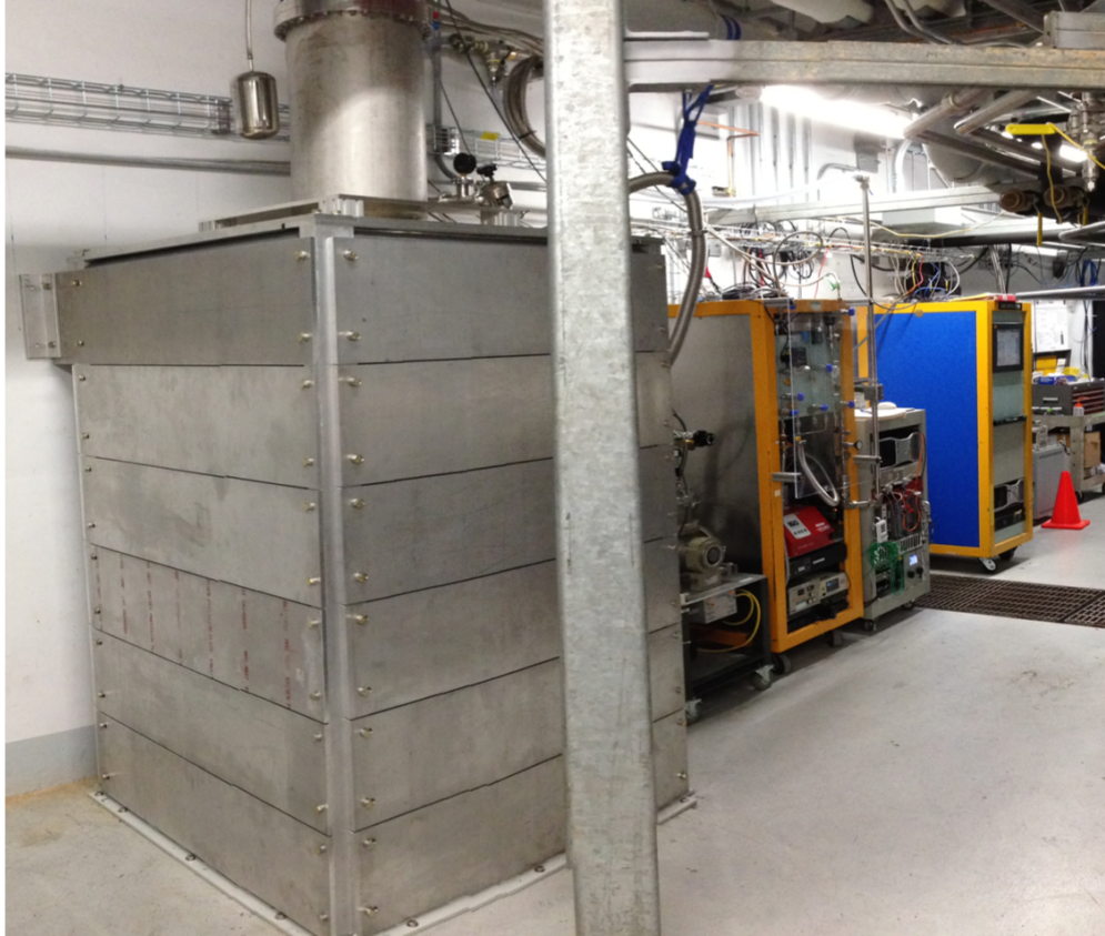
Figure 3.8: The CENNS-10 detector and all components installed in Neutrino Alley. The shielding structure can be seen around the detector along with the associated systems for the vacuum pumps, gas handling rack, fast and slow DAQ, and the cryocompressor.
