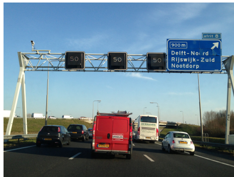
Fig. 1. VSL implementation on A13. Delft, The Netherlands.
