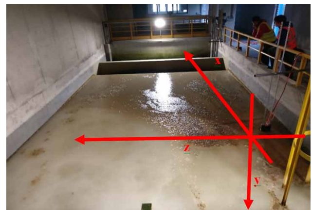
Figure 4 | Schematic of the measurement campaign with the directions at the DAF utility.
