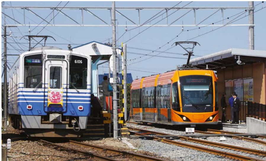
The Utsunomiya project has successfully integrated light rail with conventional rail operation.
