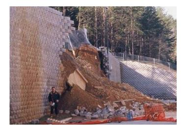
Figure 1.4: MSE wall collapse [40]
