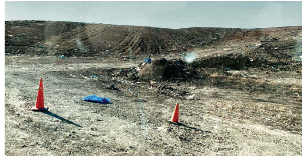
[4] MSL Sanitary Landfill with soil as daily cover material: Salina City Landfill, Salina, KS (Zhong 2019).
