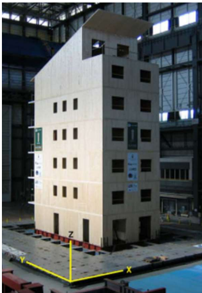
A) Test building
