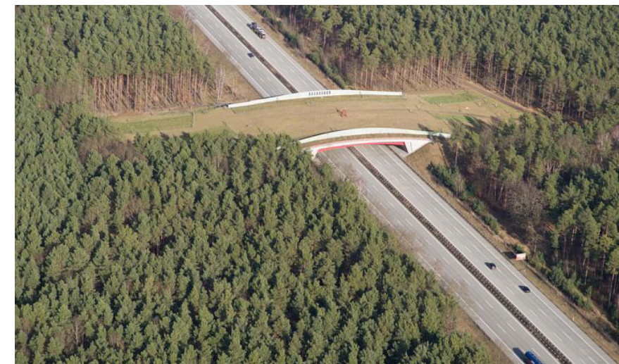
Figure 2.6: A simple thing like a land bridge that allows animals to cross over a road that run through their habitat can minimize the effects of fragmentation (Reza 2017).
