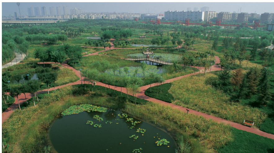
Figure 2.8: Tianjin Qiaoyuan Wetland Park was strategically designed to collect rain water to irrigate the vegetation that remediates the soil on the site. While at the same time paths and bridges frame the landscape and provide human access to this functioning wetland (Landezine/Turenscape 2011).
