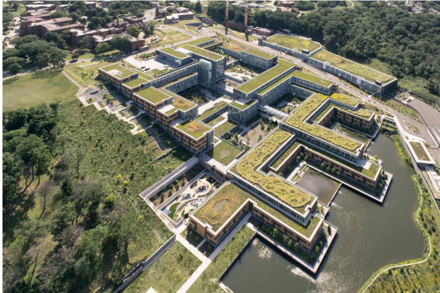
Figure 2.4: The US Coast Guard Headquarters in Washington D.C. is a great example of creative fitting. While this large building is interrupting this natural site it has one of the biggest green roofs in the world, which allows the site to maintain many of its original functions (Architect Magazine/Perkins and Will 2016).
