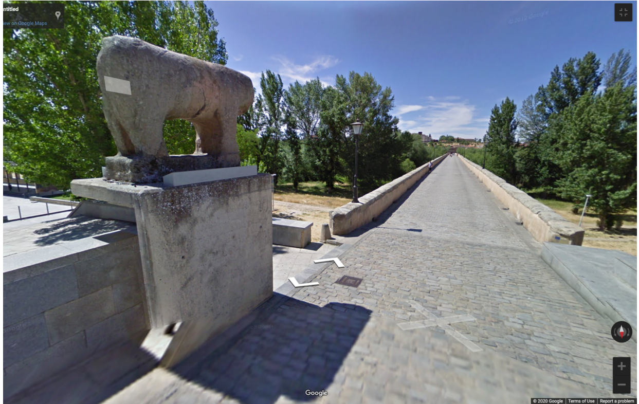
Figure 5: An example of the maximized 3D Image of the bridge over the river Tormes, Students can examine the statue of a bull and even use the arrows in the image to move across the bridge just as Lázaro does in the narrative.
