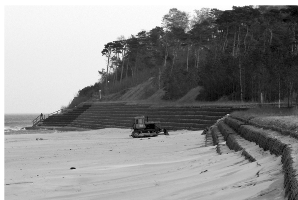
Fig. 4. Coastal protection works – seawall construction and beach nourishment
