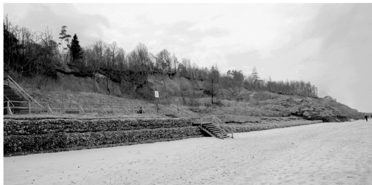
Fig. 7. A view of the landslide in 2011
