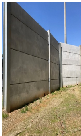
b) Precast Concrete Panels
