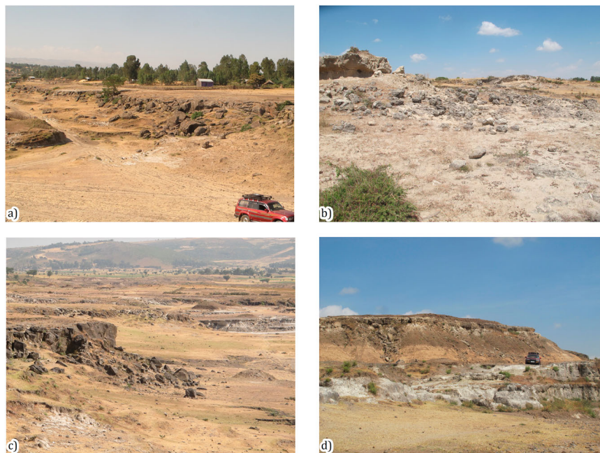
Figure 7. (a), (b), (c) Rockfalls Tuka Meja drainage banks, and (d) Translational rock slide.
