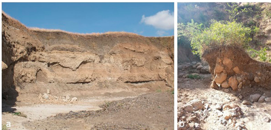
Figure 5. Bank erosion (a) Tuka Meja drainage (b) Godeti drainage.
