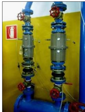
Fig. 2.16 – Laminar Flow Meters, P7205 (left) and P7209 (right)
