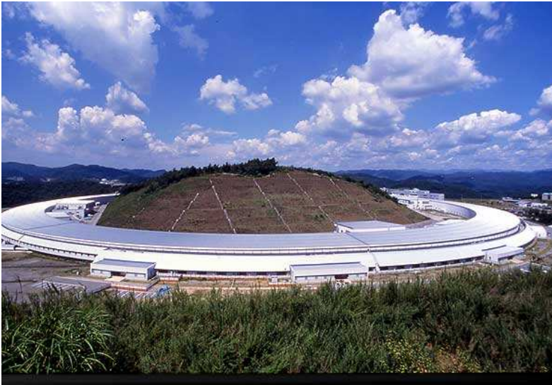
Figure 9.10: Aerial view of the SPring-8, the world's largest 3 rd generation synchrotron light source. Credits: JASRI.
