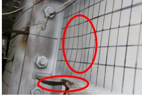
(a) Significant local buckling deformations at 0.05 rad
