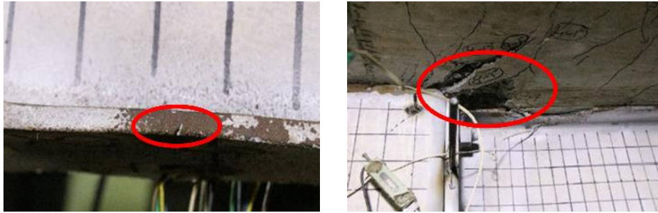
(b) Bottom flange cracking and concrete crushing at 0.06 rad
