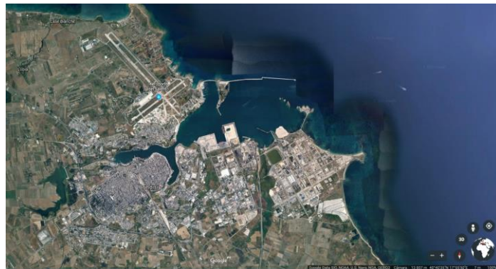
Fig. 63. The harbour of Brindisi in modern times. One can observe it retained its protected shape and the current subdivision between several sectors of the outer harbour (including the two modern cutwaters) and the inner harbour, smaller and more sheltered. Nearby, the Lago di Cillarese; ancient sources do not mention channel connections in the same pattern as that of Lakes Auernus and Lucrinus, but this could potentially have been used as a location for ship storage, even without channel construction.
