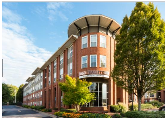
9. Atlanta Apartment Building
