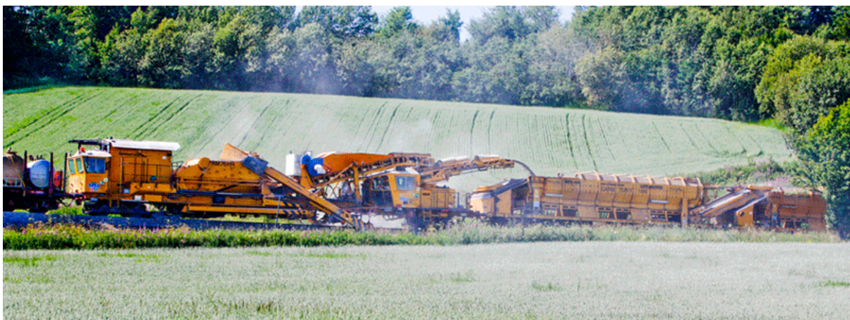
Figur 15 – Ballastrensing. Foto: Baneservice 29
