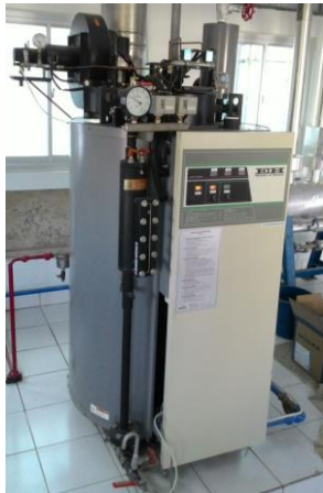
Gambar 2.1 Boiler Miura EH-500 F Gambar 2.2 Bagian-bagian boiler compact secara umum
