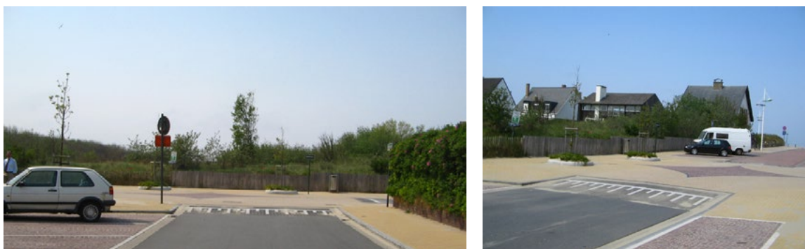
Fig. 7. & 8. Zeebrugge, Belgium. The surface of the intersection is elevated to the level of the pavements and integrated with their surface. Source: photo by Hubert Trammer, May 4 th , 2007.
