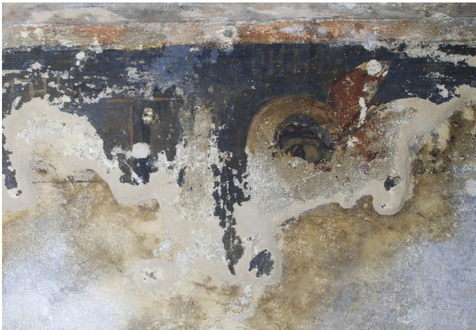
Fig. 5 and 6 Ottoman vs Christian traces of paint and coatings: searching for evidence to solve issues of interpretation, Tower of the Winds (photo credit: Greek Ministry of Culture & Sports - Fund of the Archaeological Proceeds)
