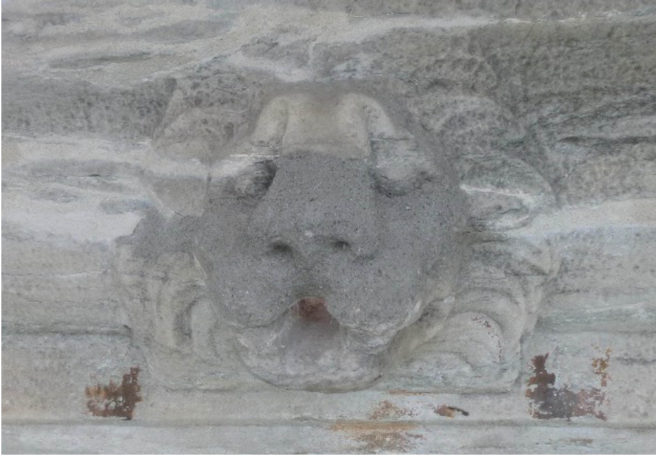
Fig. 4 Preservation of a lion's-head addition which helps rainwater drainage from the roof, Tower of the Winds (photo credit: Greek Ministry of Culture & Sports - Fund of the Archaeological Proceeds)
